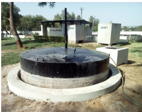
Fig. 2 Dairy effluent scum based biogas plant at M/s Vidya Dairy, Anand
